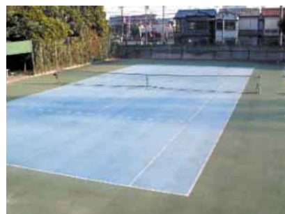
Tennis courts using recycled polyurethane, in Nagoya Works
