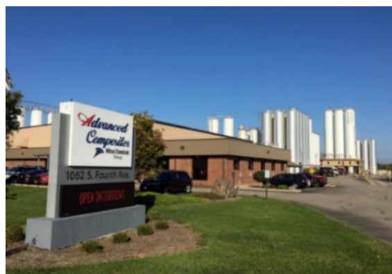
New facility site at Advanced Composites, Inc.
