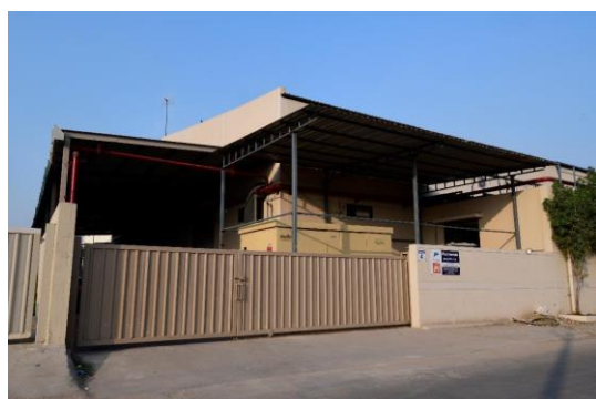
Testing lab exterior
