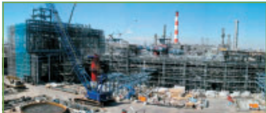
3 EPT (Under construction)
